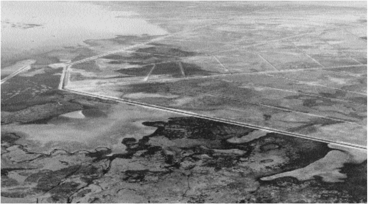
South-east part of Yay Lake and Camiz Lake Pump Station (by U. Ozesmi)
